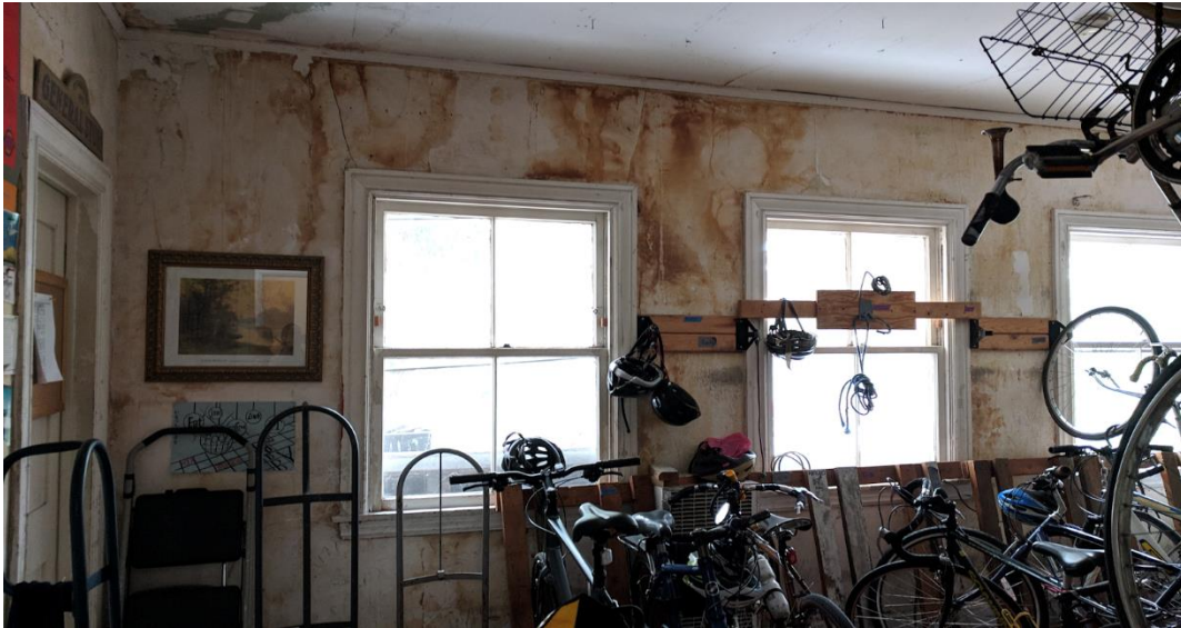
Figure 5.2. Original condition of LA Eco-Village building as seen in the bike room.
